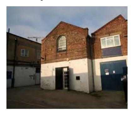
A tight-knit group of buildings off Sugar House Lane, two and three storeys in height, built with red brick with characteristic industrial detailing, such as the bullnose engineering bricks which are used for the window cills.
