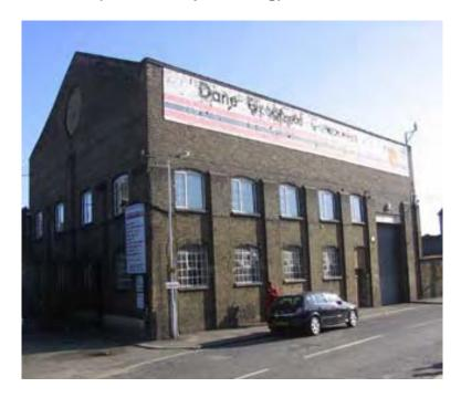
Built around 1900, 7 Sugar House Lane is solidly constructed in London stock brick and occupies a prominent position on the bend of the road. It is six bays wide, including a double height loading bay, with small pane steel windows on the ground floor. The upper windows are modern replacements.
