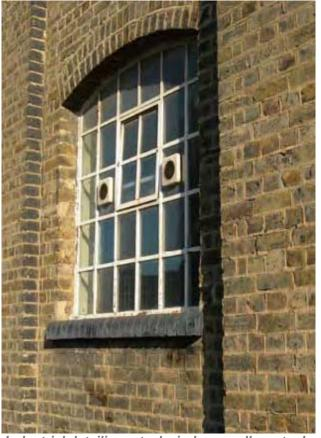
Industrial detailing: steel windows, yellow stock brick with bullnose engineering brick cills
