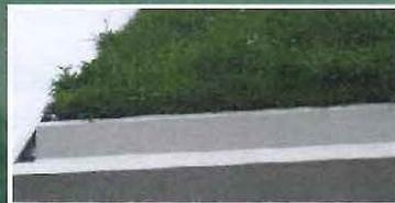
■ Engineered metal L shaped retaining profile
