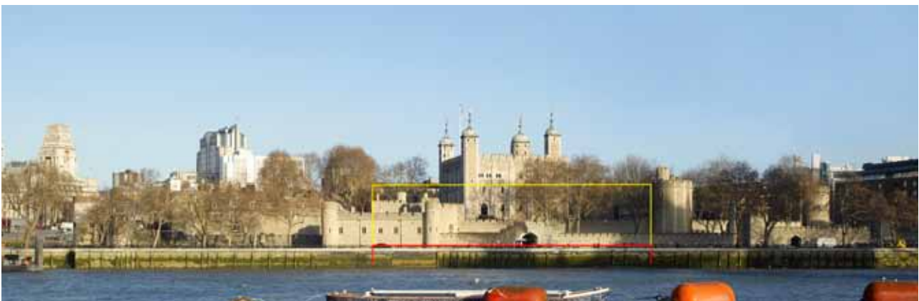
Telephoto view of Protected Vista from Assessment Point 25A.1 to the Tower of London
