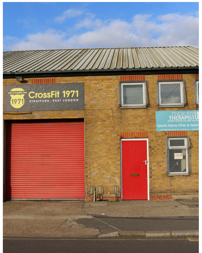
Sports facilities and associated services offered in industrial units neighbouring central Stratford.
