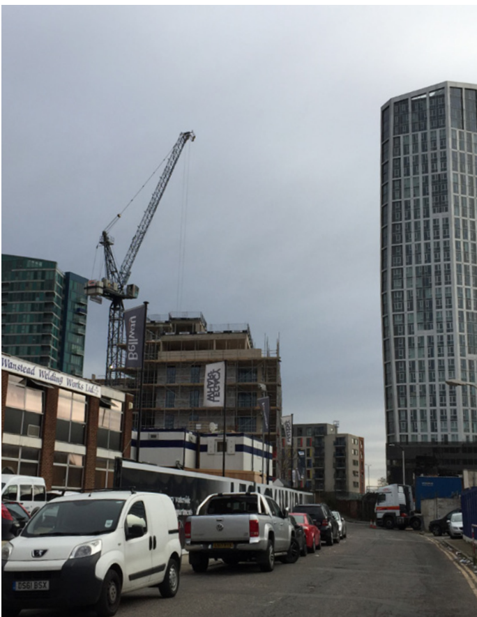
Large-scale residential-led schemes alongside older industrial building stock.
