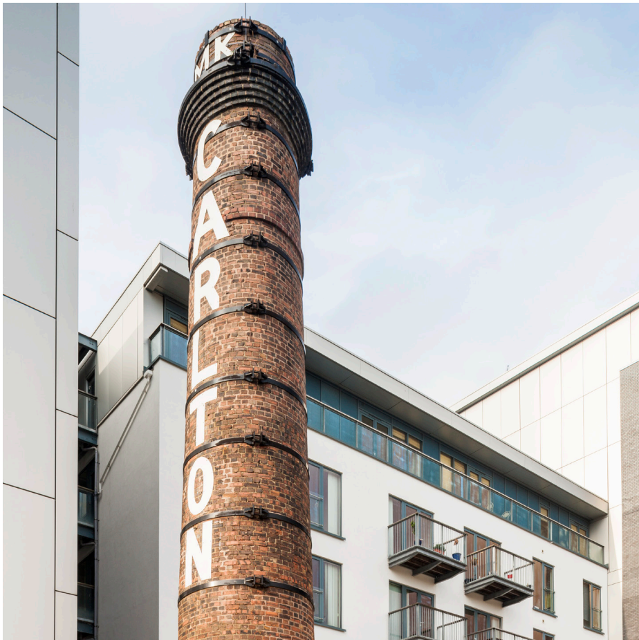
Above: Crown Wharf chimney stack
