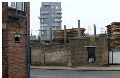
Boundary Wall to the former Hope Chemical Works
