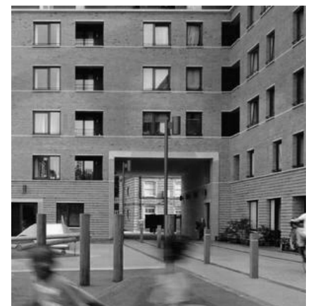
Peabody Avenue, Pimlico, London, Haworth Tompkins : The internal yard is connected to the street by a double height opening through the building
