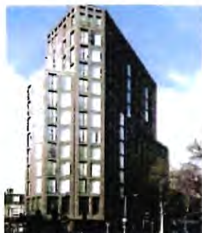
Sculptural massing form (H10 Hotel, Southwark - Maccreeor Lavington Architects)
