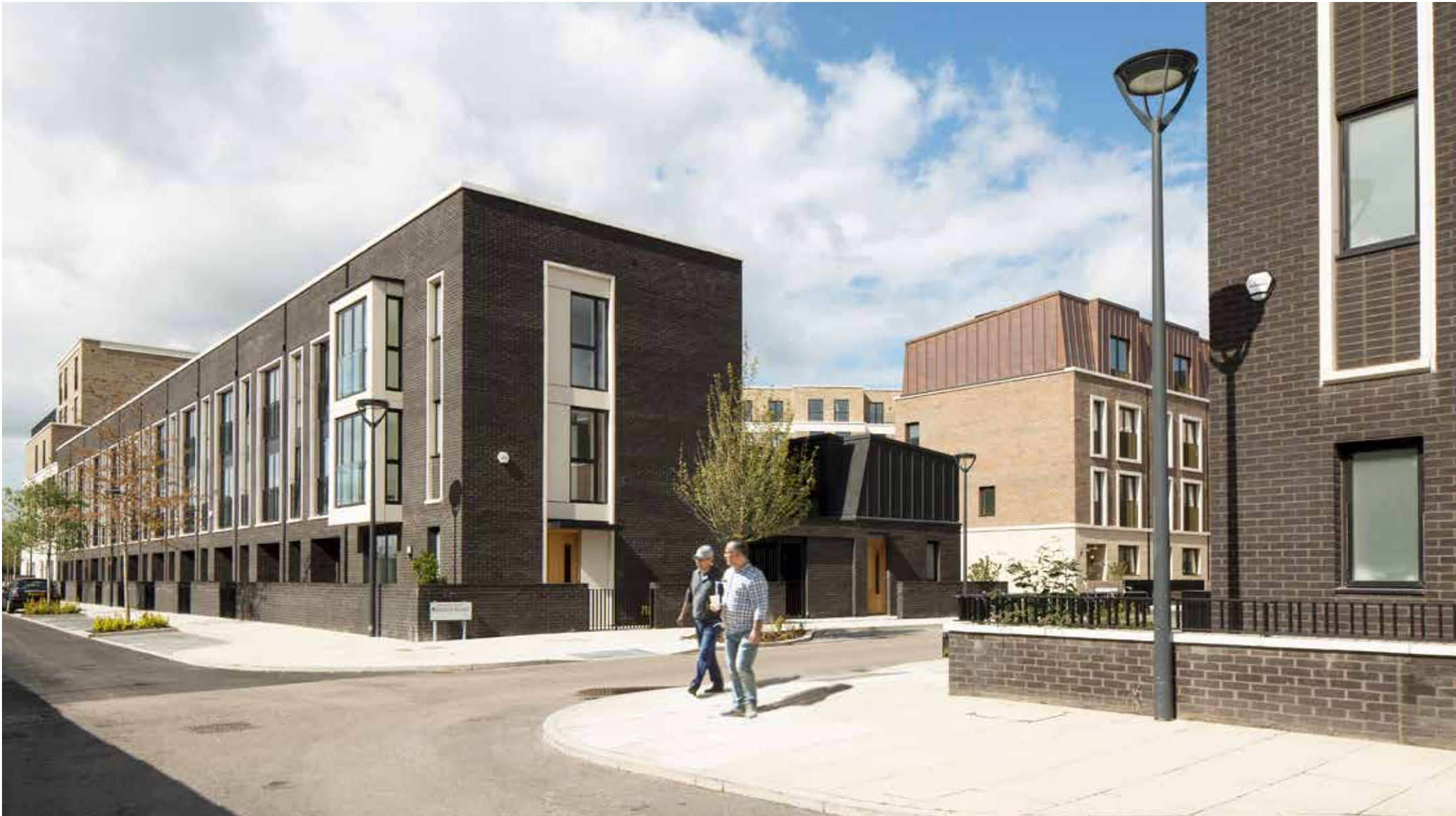
The form of the building manages the transition at the junction of street with The Green. Defensible space is clearly defined by simple brick walls, with a simple materials palette, front doors, fenestration with feature surrounds and oriel windows providing activation and interest to the street scene.
