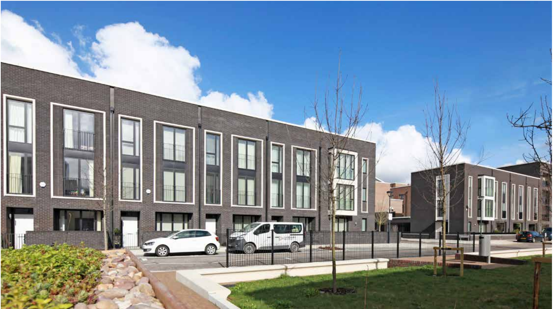
View of the emerging street scene at Chobham Manor. The Multi Generation Homes complete and bookend the run of townhouses to The Green. Full height openable windows at ground level and oriel windows above provide panoramic views from the family kitchen, living space and master bedroom across The Green which is the heart of the development.
