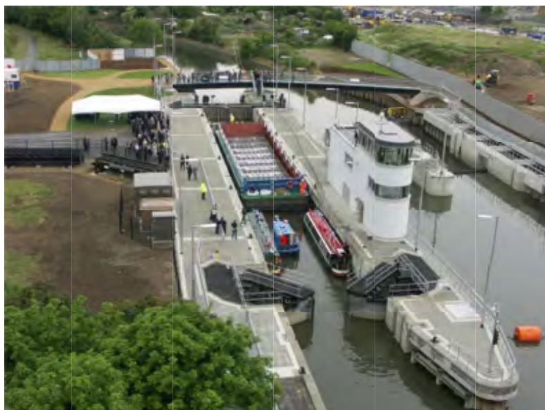
Figure 12 - Three Mills Lock
