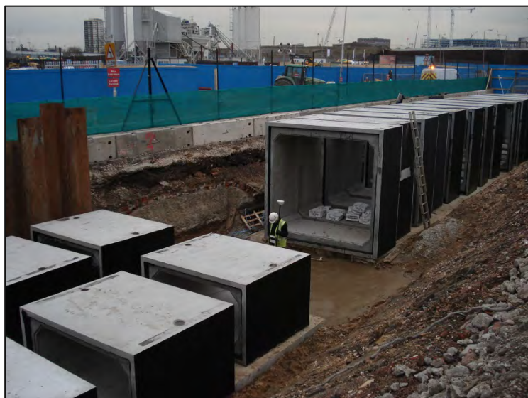
Figure 20 - new culverts ready to be placed (May 2009)
