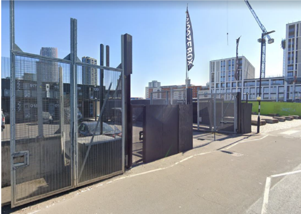
Figure 5: Existing gate in public highway
