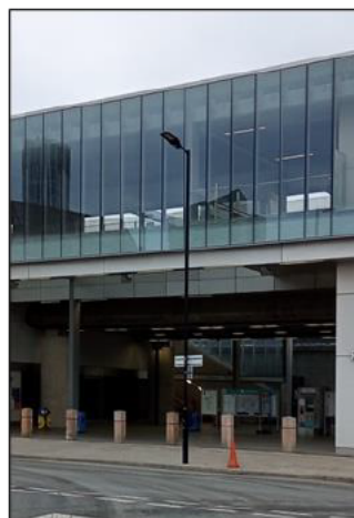
Figure 9 – Lighting column outside Pudding Mill Lane DLR station
