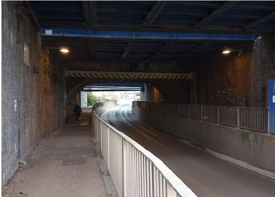
Figure 11 – Site Photo of Marshgate Lane Underpass – Northern Portal Looking South
