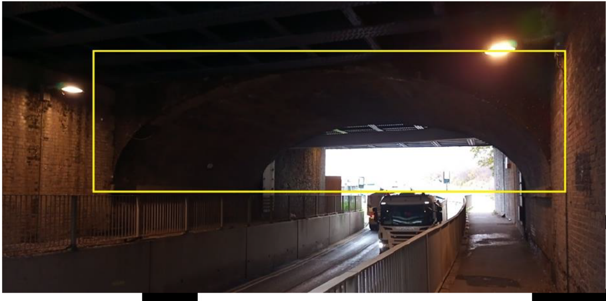
Figure 16 – Photo Highlighting the Arch underpass southern portal looking north
