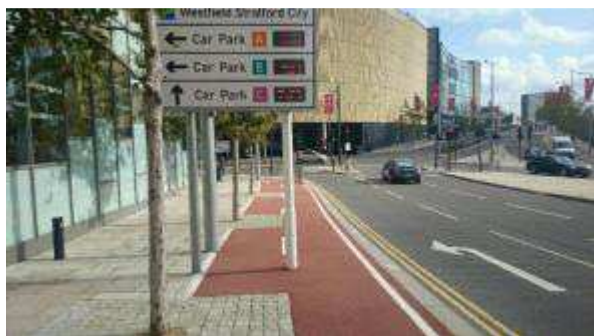
Figure 2.3: Poor Quality Cycle Infrastructure – Westfield Avenue
