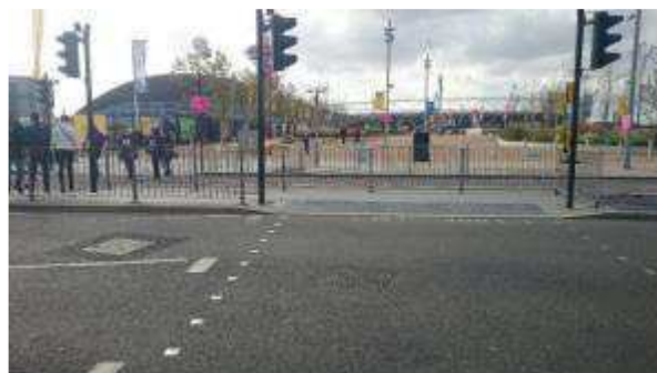
Figure 2.4: Indirect Pedestrian crossing – Westfield Avenue
