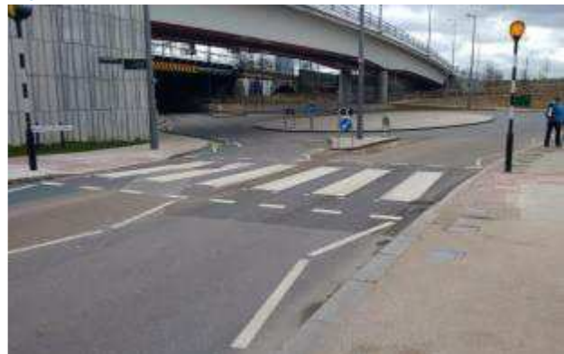
Figure 2.11: Warton Road Roundabout
