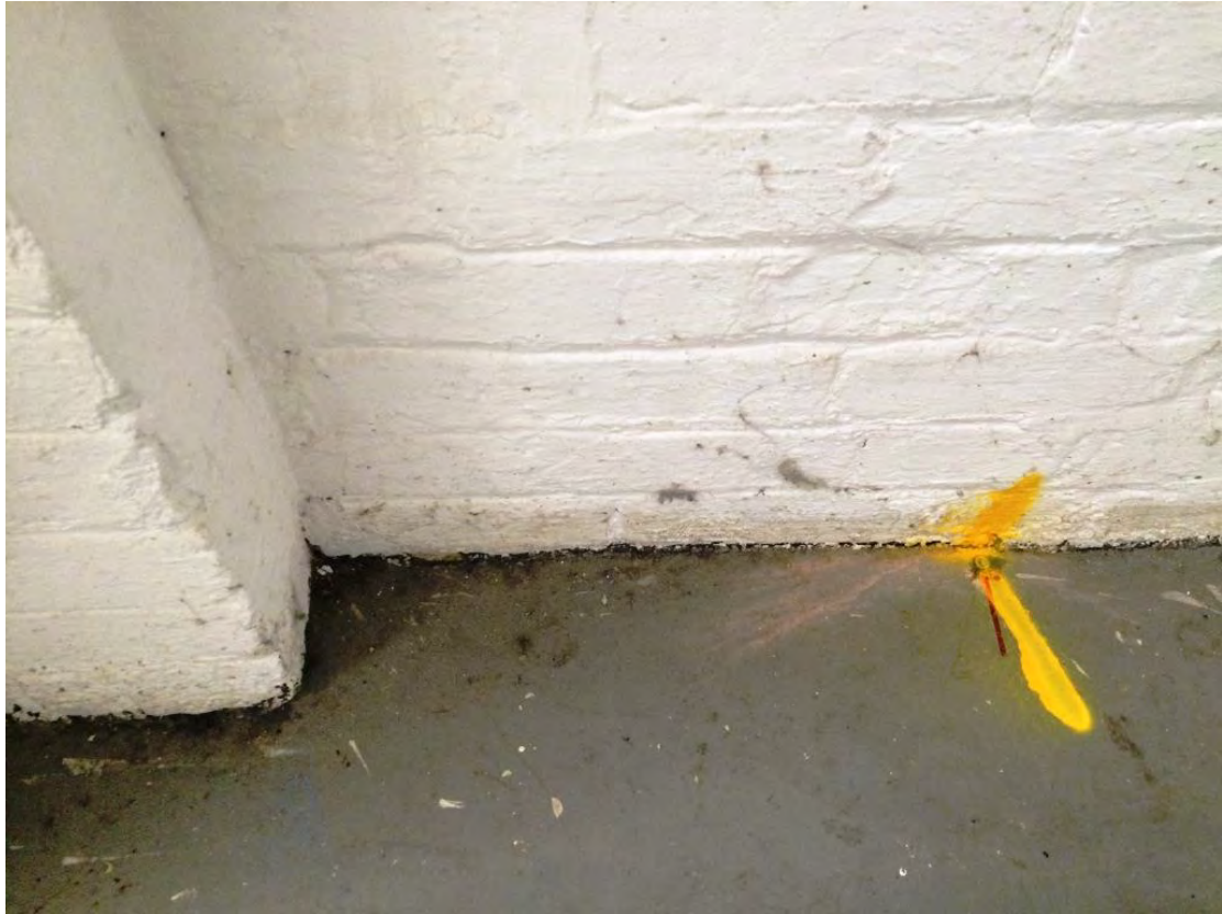
Point 17 – (facing West) 0.53m North of wall corner (537335.16, 184159.67)
