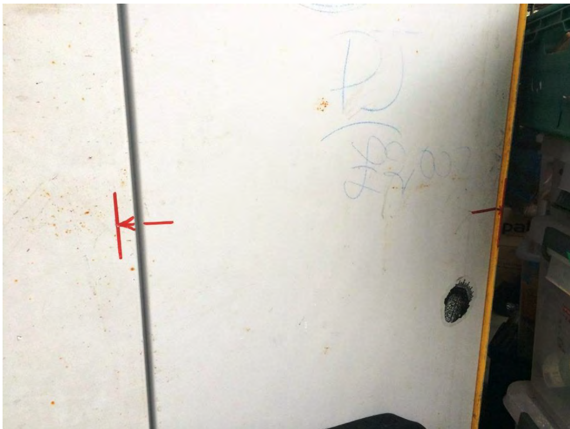
Point 9 - (facing South East) 0.63m North from angle iron wall end (537327.59, 184158.20)
