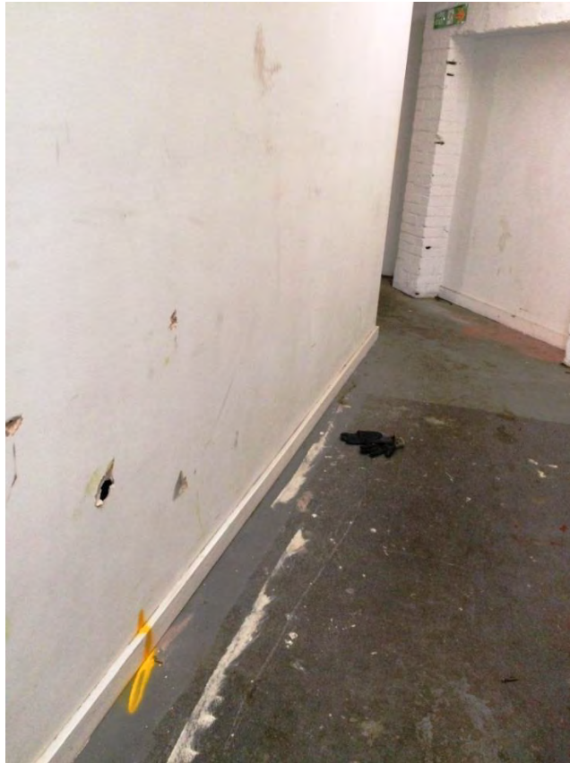
Point 21 – (facing West) 3.00m East of wall corner (537340.53, 184160.72)
