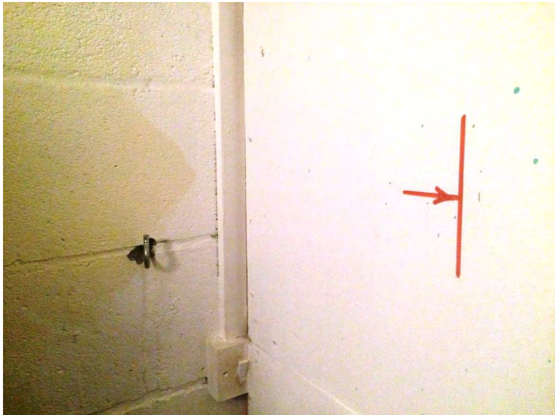
Point 6 – (facing South West) 0.40m North of internal wall (537314.98, 184155.73)
