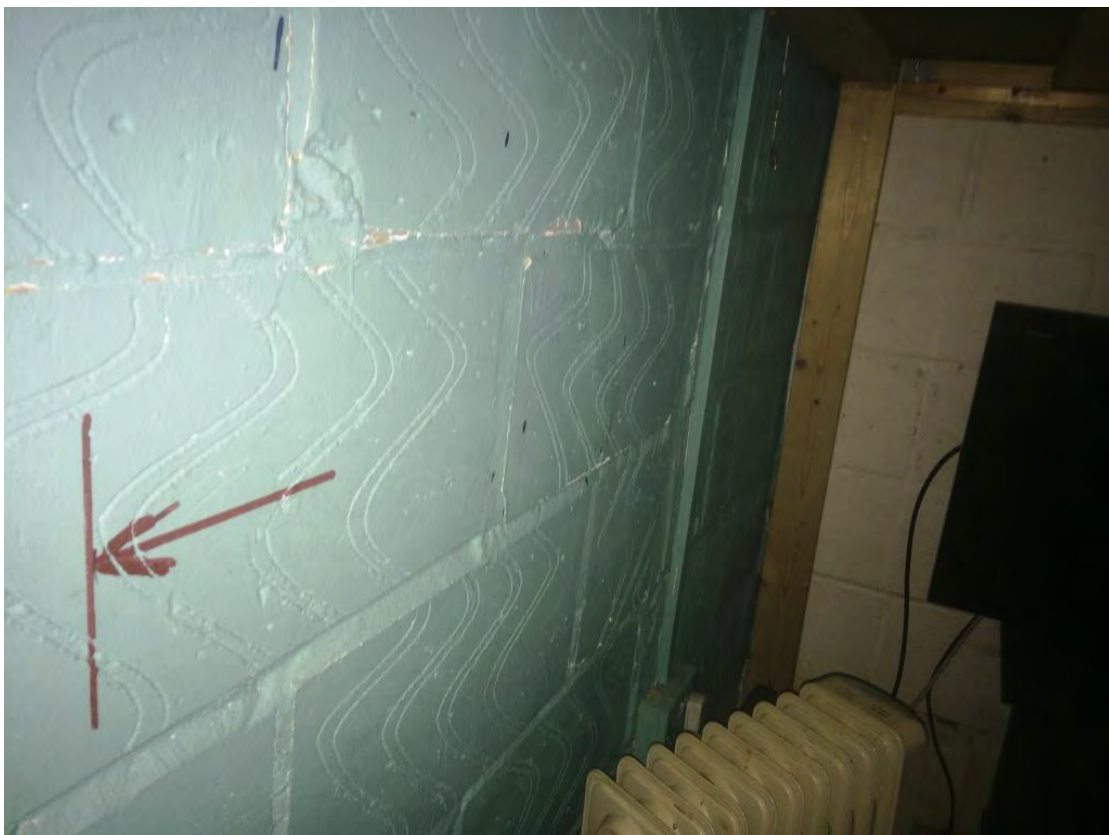
Point 7 – (facing South East) 1.60m North of internal wall corner (537319.51, 184156.62)
