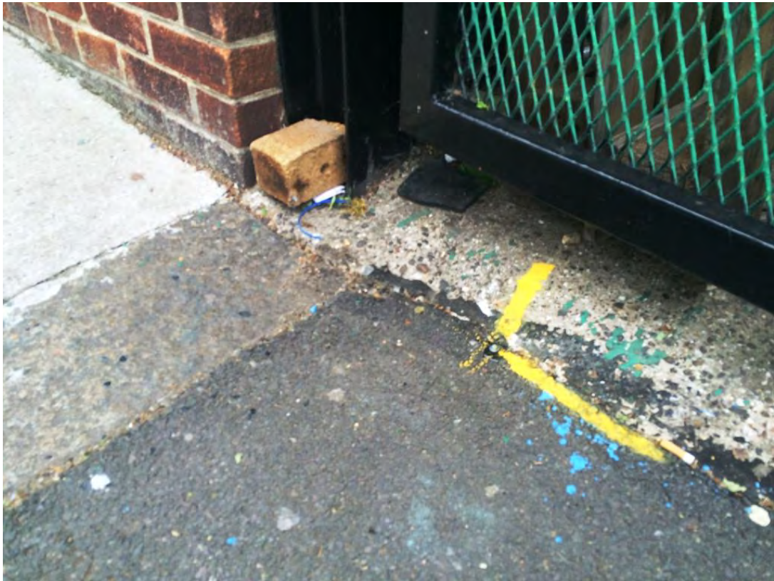
Corner point (facing North East) – 0.50m south of building corner (537305.42, 184153.86)
