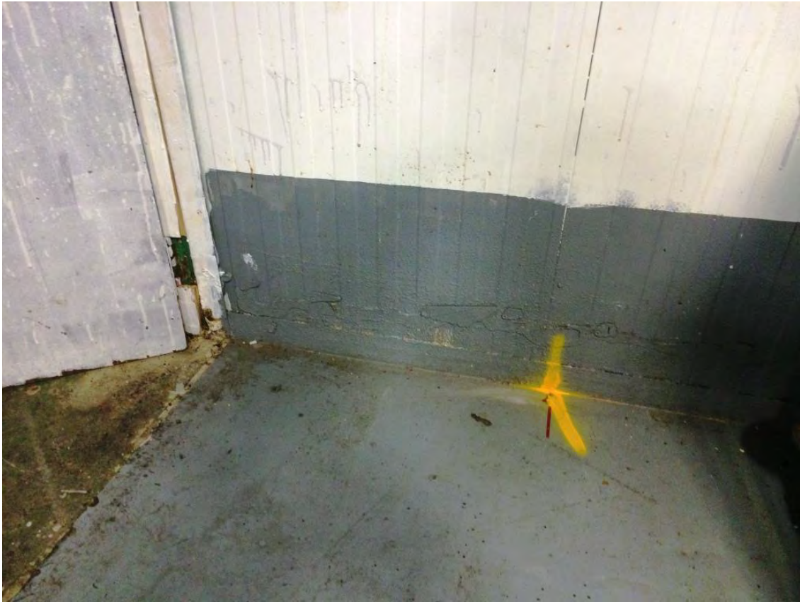
Point 10 – (facing West) 0.65m North of angle iron wall end (537327.69, 184158.22)
