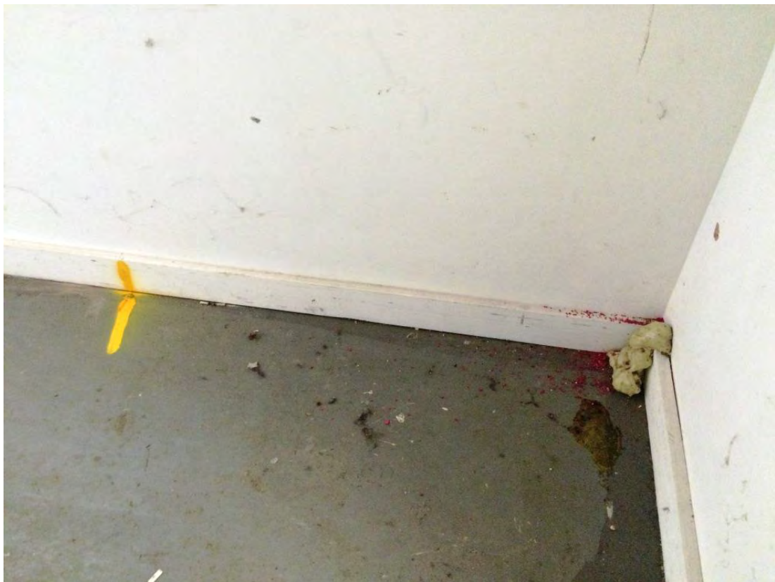
Point 18 – (facing East) 1.11m North of internal wall corner (537337.48, 184160.13)
