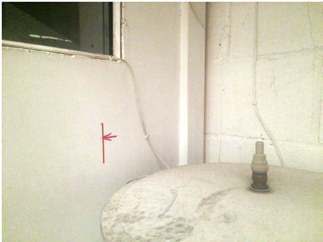
Point 5 – (facing South East) 0.39m North of internal wall (537314.88, 184155.71)
