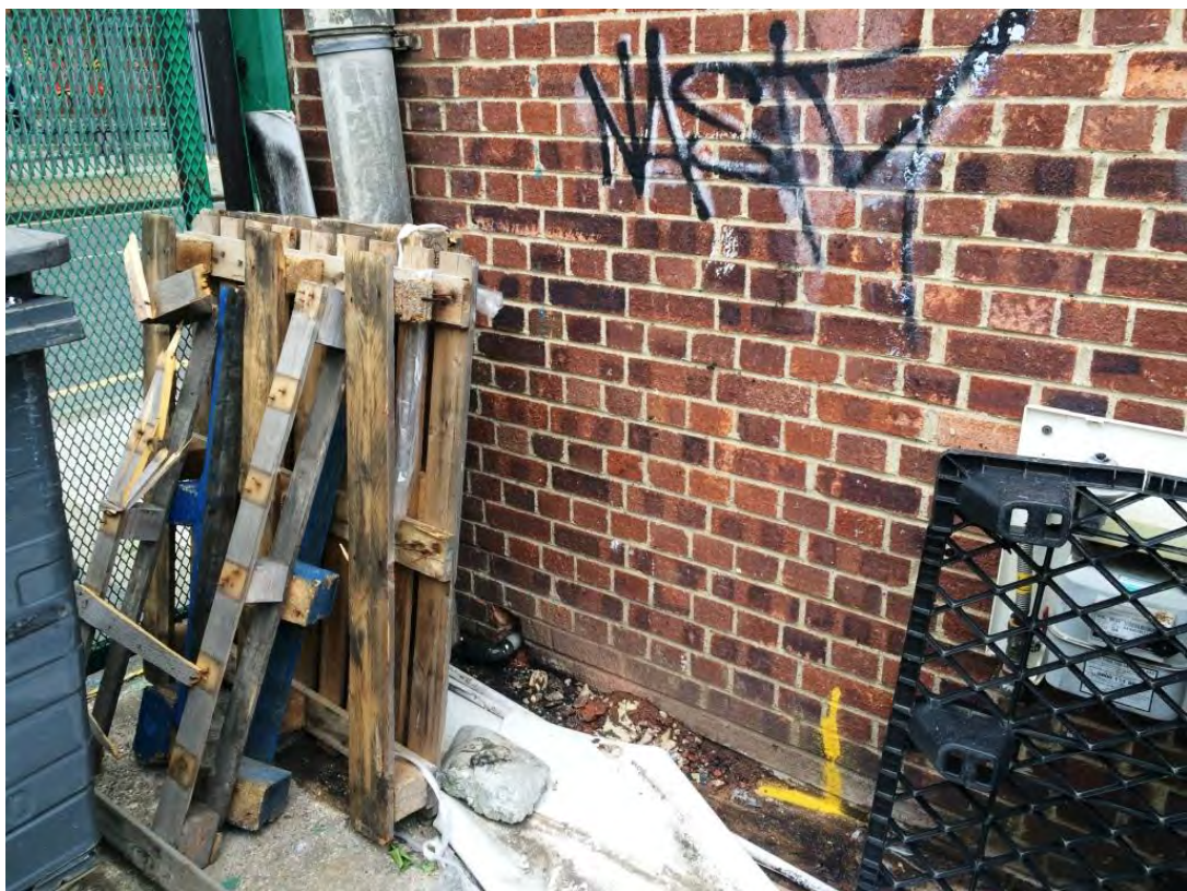
Point 1 (facing North West) – 1.80m East of building corner (537307.26, 184154.22)
