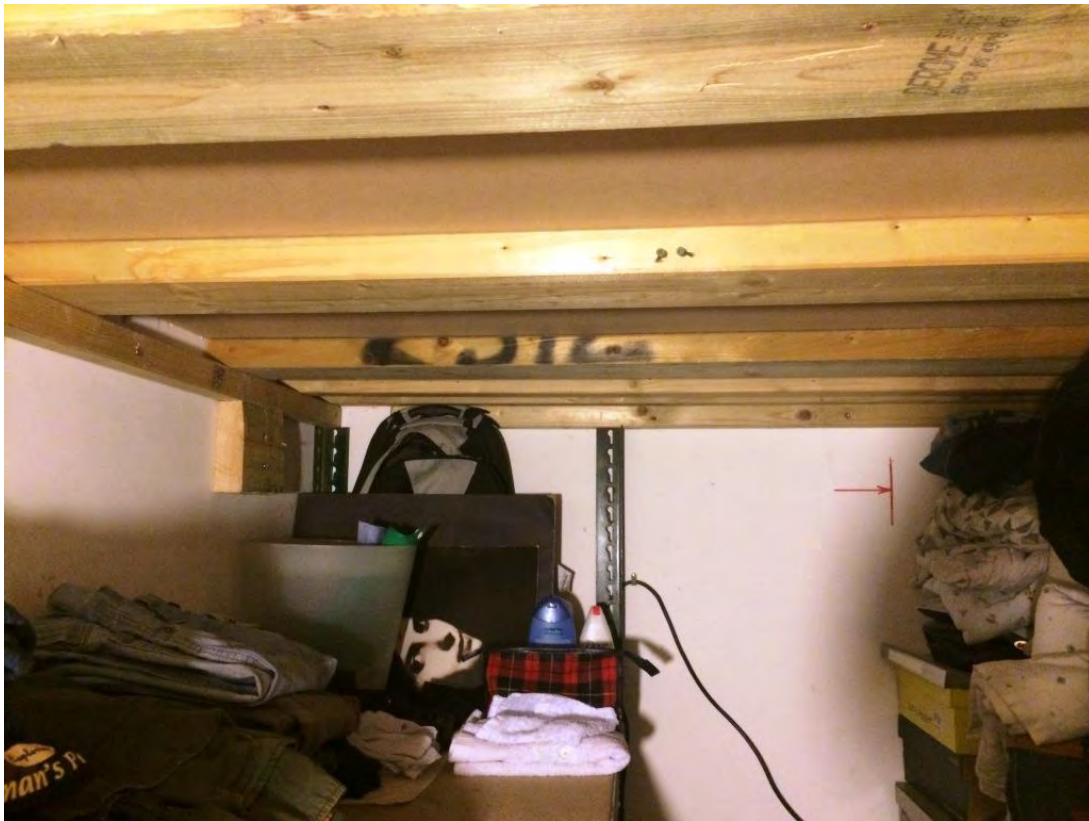
Point 19 – (facing West) 1.16m North of wall corner (537337.61, 184160.16)
