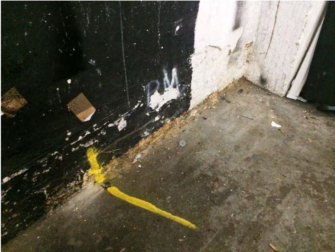
Point 12 – (facing North West) 0.85m South of wall corner (537335.33, 184159.71)
