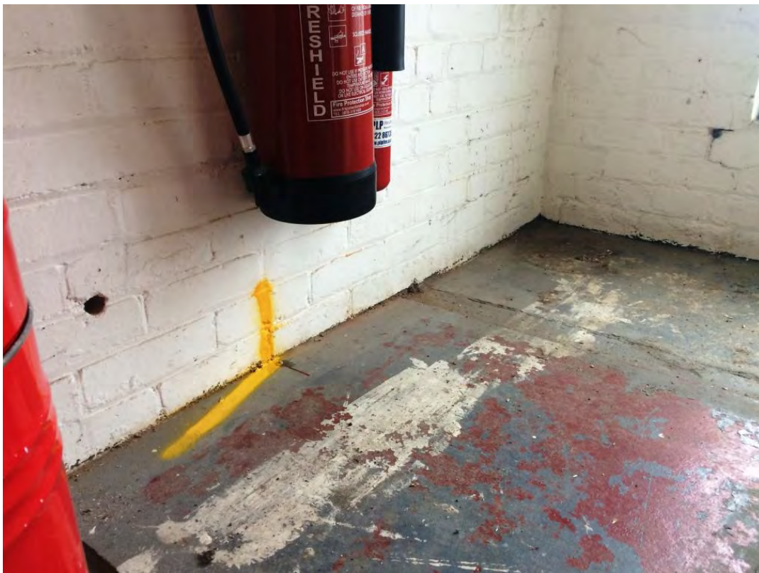
Point 22 – (facing North East) 1.15m West of wall corner (537347.48, 184162.08)
