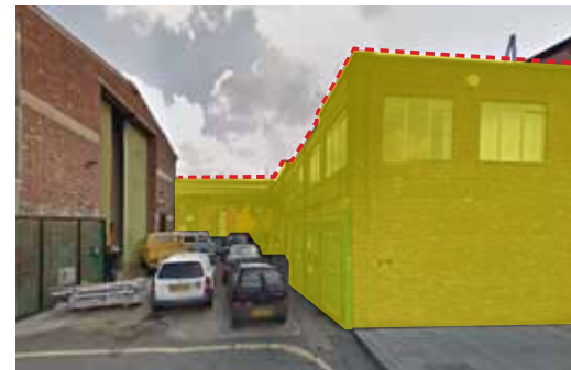
2. Part of Vittoria Wharf to be demolished under proposed option
