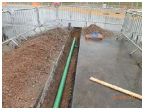
New ducts installed above Marker Layer
