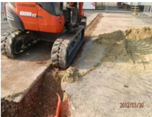
Reinstated marker layer when penetrated
