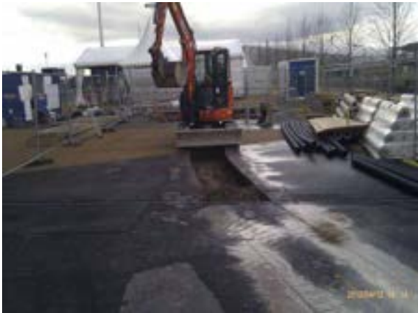
Excavation above marker layer
