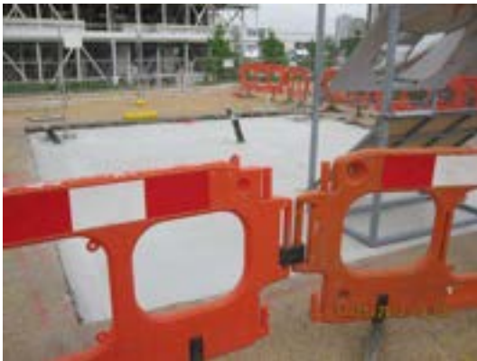
Concrete filled entire excavation no need for backfilling
