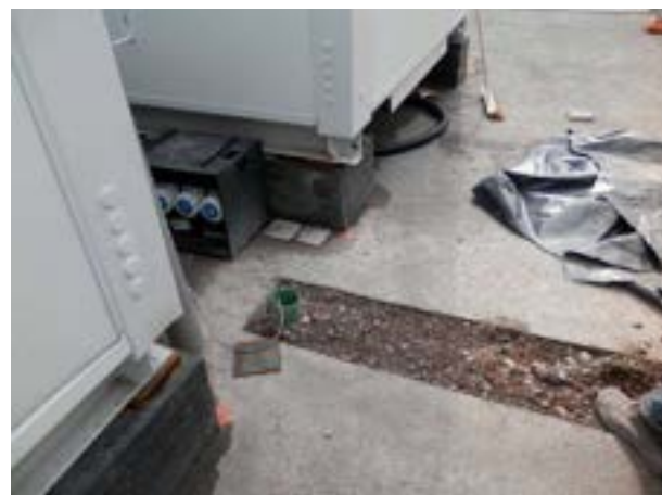
Use of reused HHL material for backfilling
