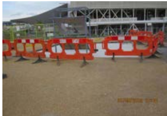
Concrete filled entire excavation no need for backfilling
