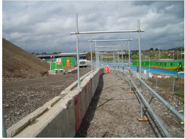
Walkway protected using VCBs and scaffold barrier
