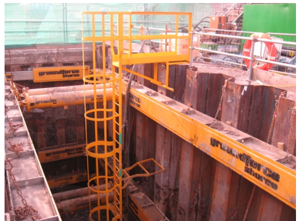
Hoop ladder access into a cofferdam
