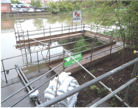
Custom built scaffold providing access to marine craft.
