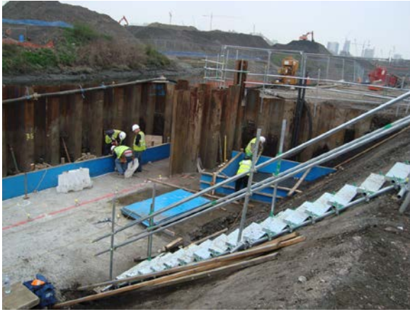
Access into a battered excavation using a self levelling staircase
