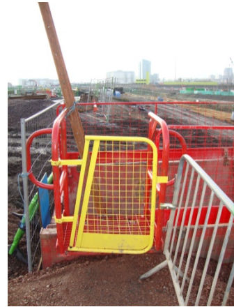
Proprietary vertical ladder system attached to a trench boxes
