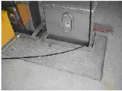
Metal Riser Flooring with 65mm perimeter upstand
