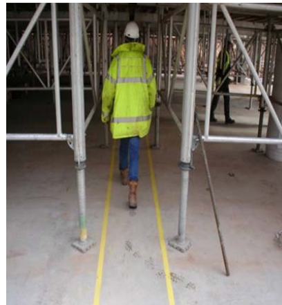
Painted lines defining a walkway
