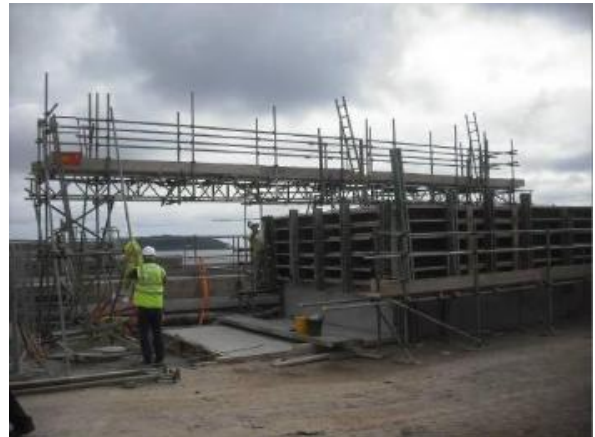
Access arrangements and guarding of exposed edges for work on shutters
