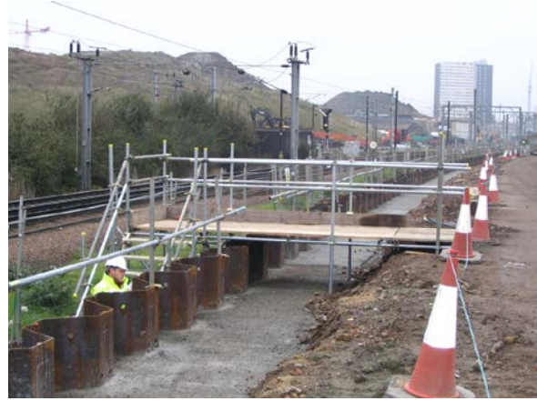
Scaffold access across a sheet piled retaining wall
