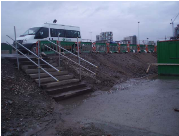
Custom built scaffold staircase
