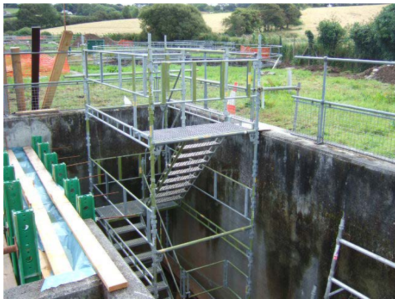
Tower staircase access into a shaft
