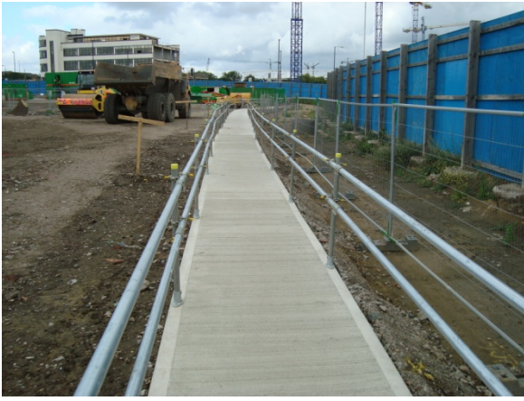
Concrete walkway with scaffold barrier
