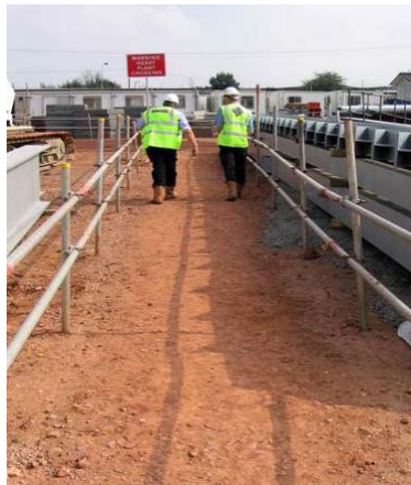
Walkway with scaffold barrier
