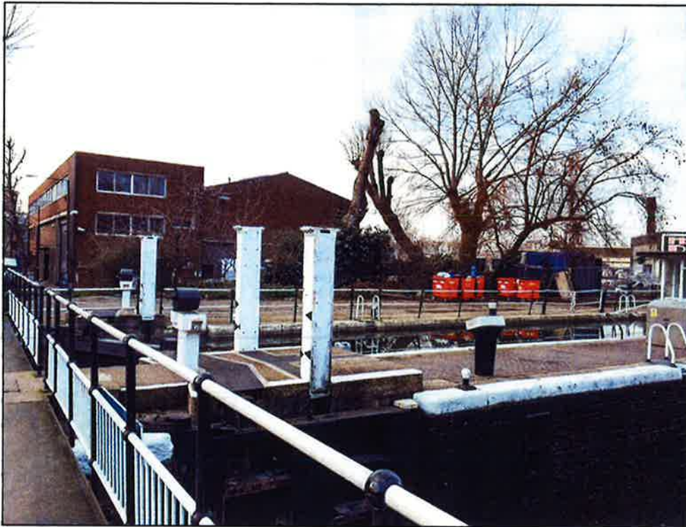
View of warehouse from Old Ford Lock
