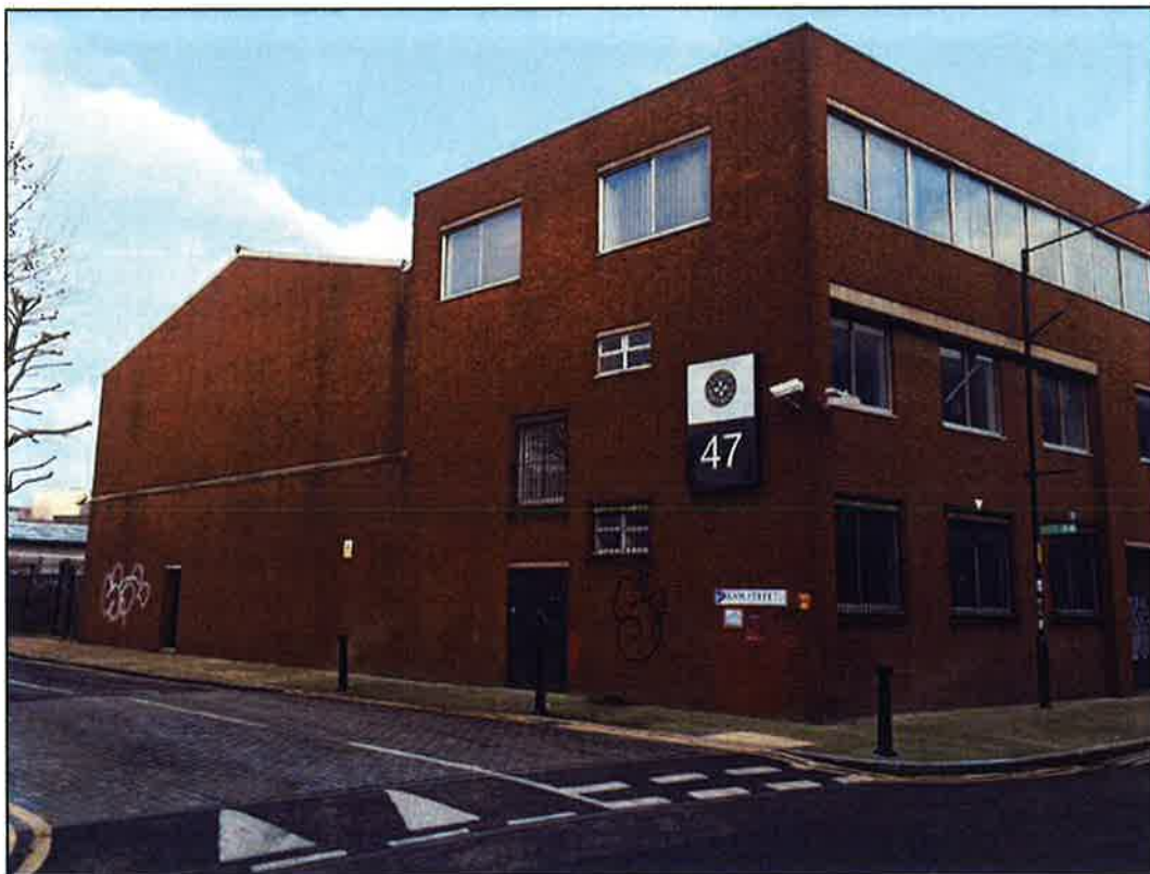
Bream Street elevation of warehouse
