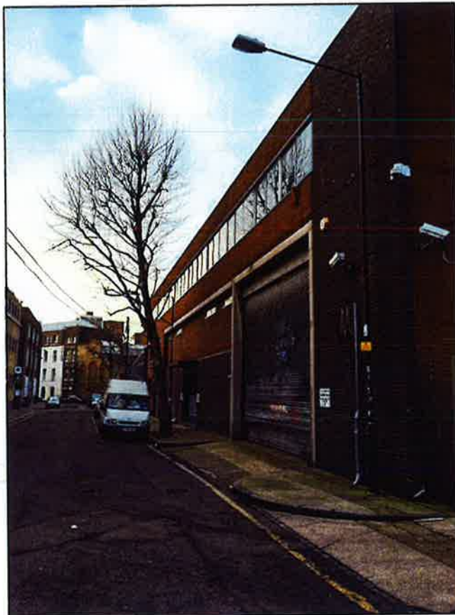
Dace Road elevation of warehouse
