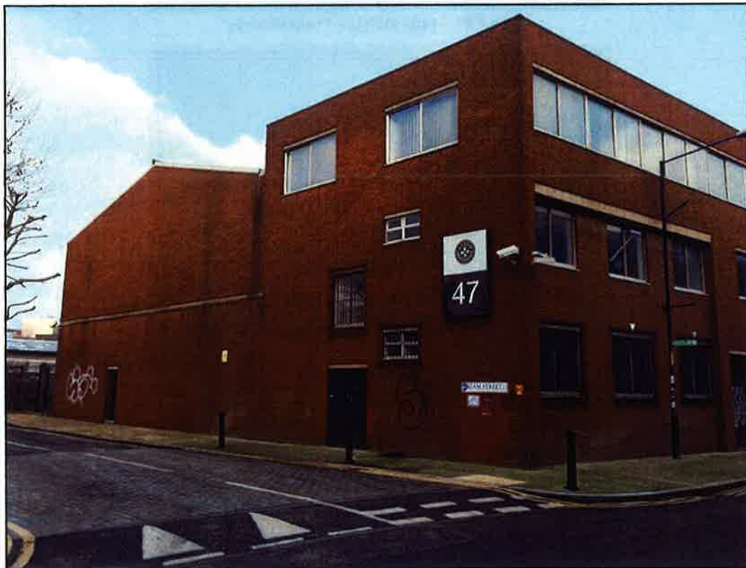
Bream Street elevation of warehouse
