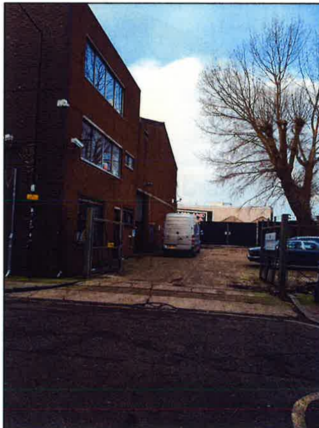
Car park to warehouse off Dace Road
