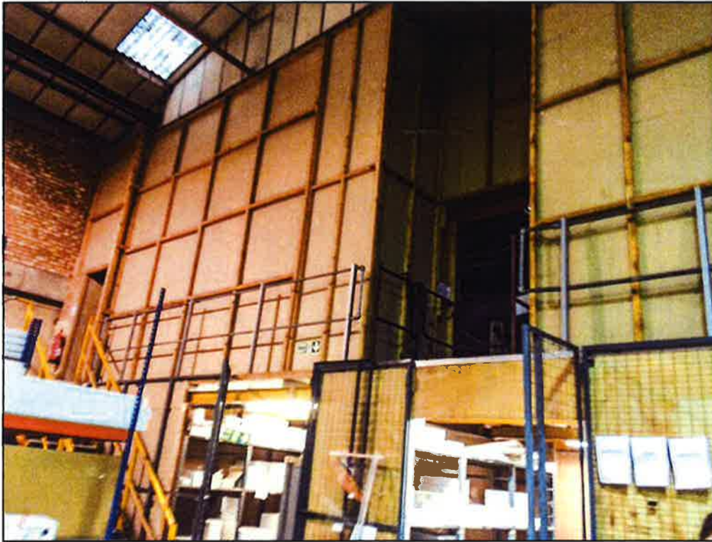
Interior of main warehouse
