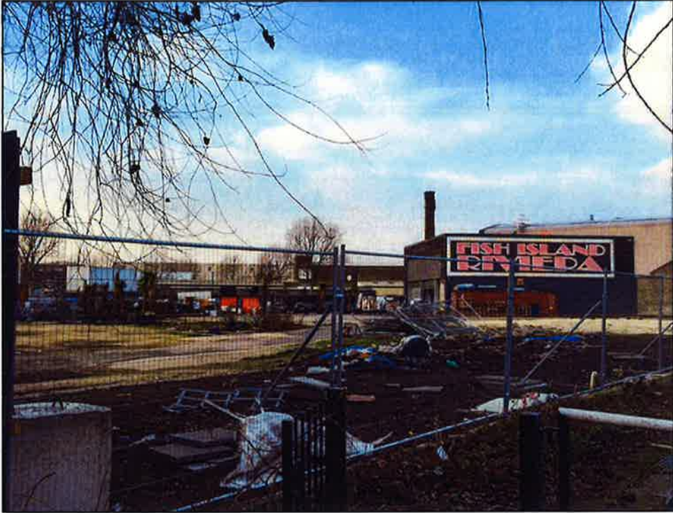
Hardstanding adjoining H Forman's warehouse
