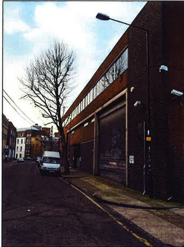
Dace Road elevation of warehouse
