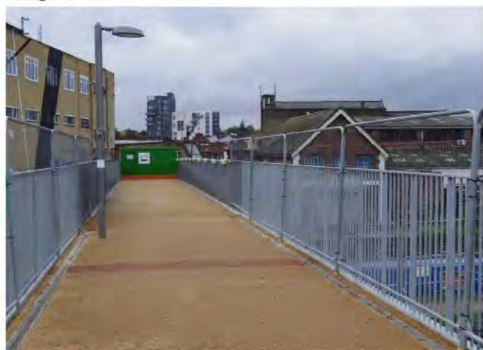
Figure 9.7 Wallis Road pedestrian bridge deck
