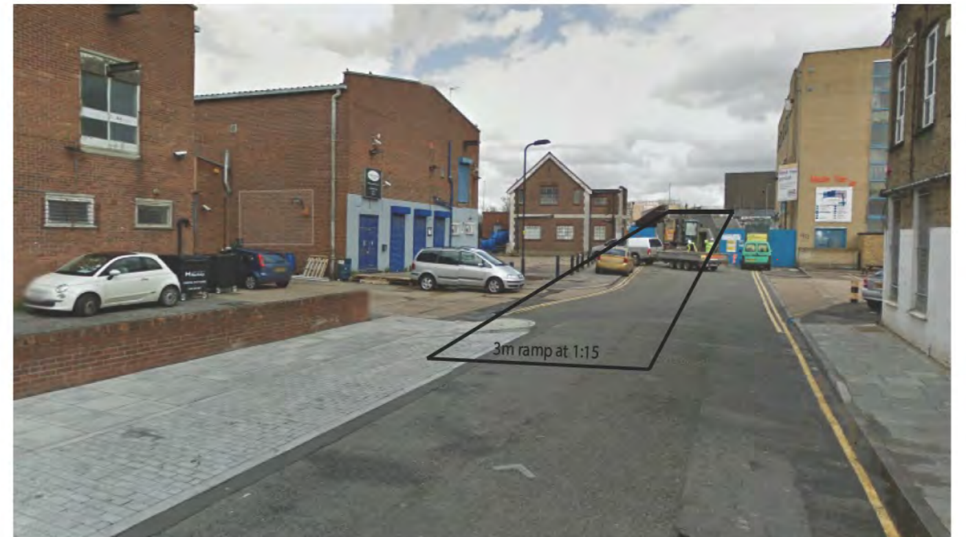
Figure 9.15 - Approximate location and size of 3m wide shared use ped/cycle ramp for option G
