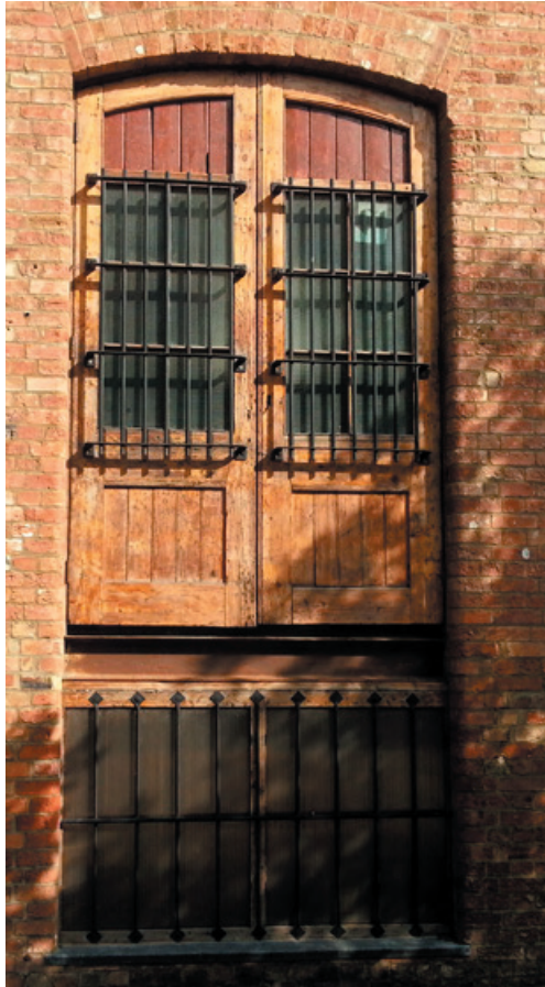
Existing loading doors to the south elevation
