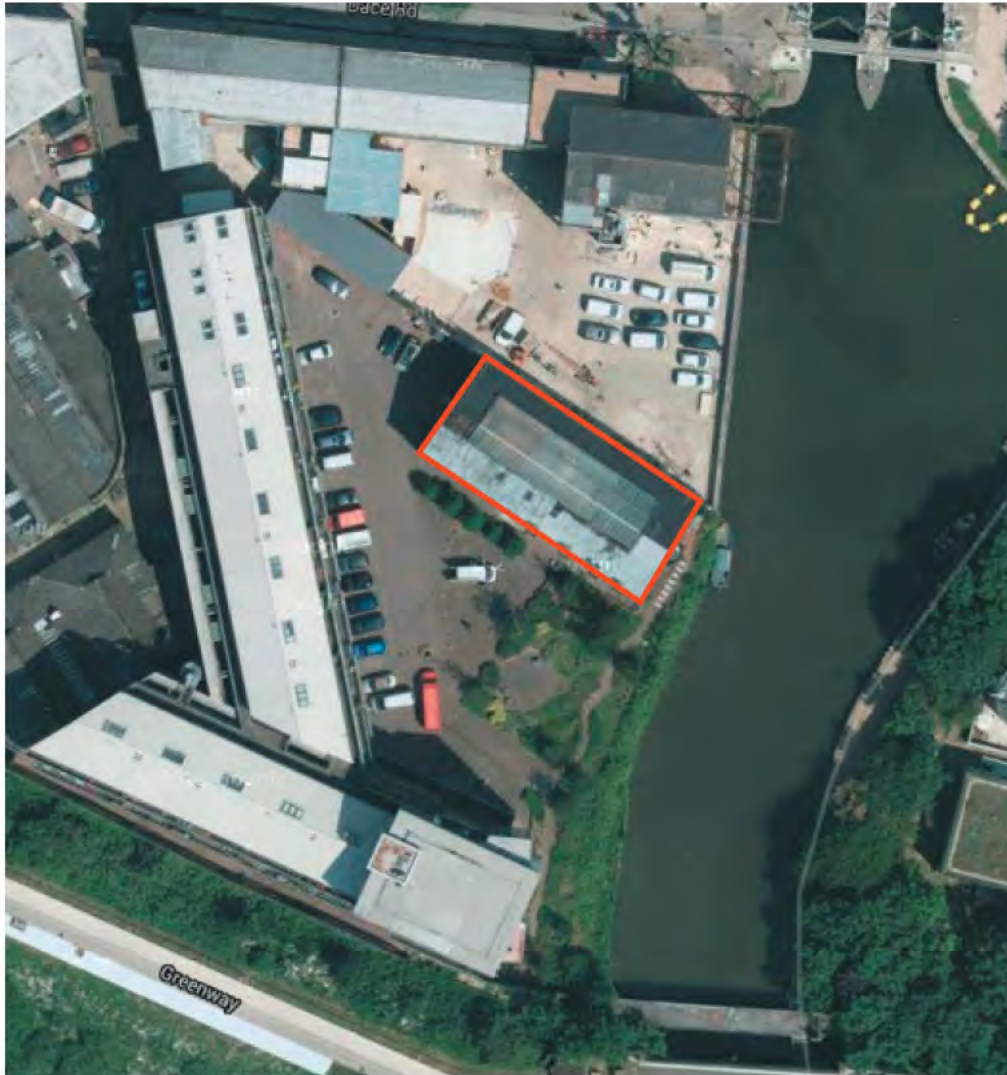
Aerial photograph with the site outlined in red
