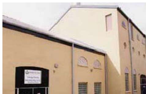
Figure 4 - Barkantine Energy Centre (courtesy of Cofely GDF Suez)
