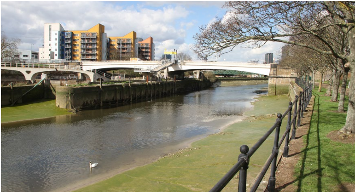
Construction of the Twelvetrees Bridge pedestrian and cycle ramp at Bromley by Bow completed in the last period, closing a major gap in the Leaway.
