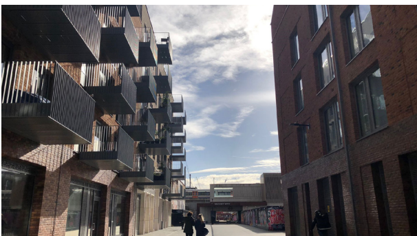
Image: Access to the station from Wallis Road
