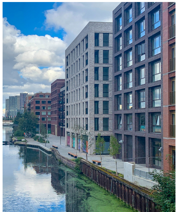
Image: Phase 3 Fish Island Village (Neptune Wharf)
