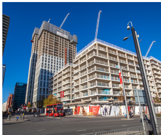
Image: Cherry Park progress on site (December 2021)
