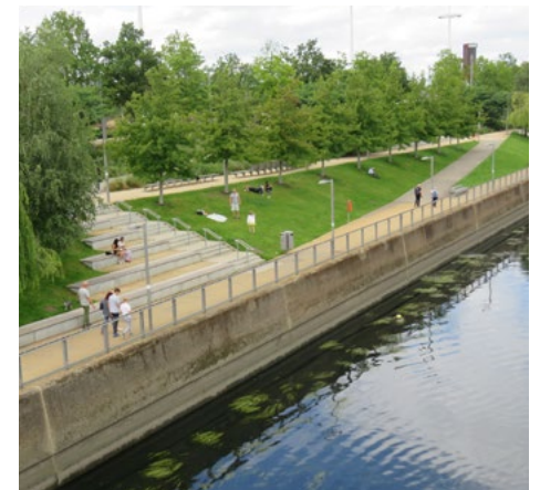
Riverside walkways and terraced seating characterises the South Park - looking towards the combined heat and power (CHP) Energy Centre
