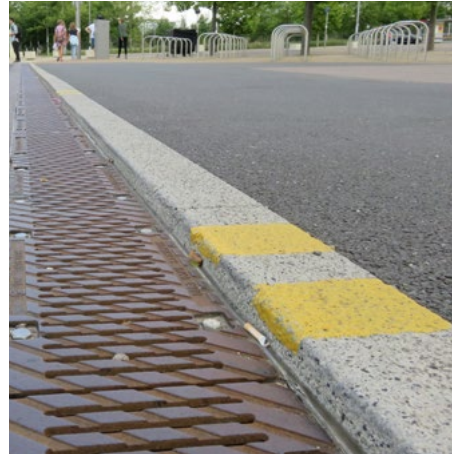
Typically all primary roads are to restrict loading at all times with double yellow blip markings.
