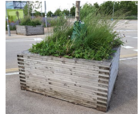
Existing timber planters - not to be specified
