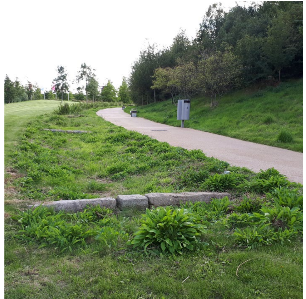
North Park - Linear swales are an integral part of the SuDS strategy at Queen Elizabeth Olympic Park
