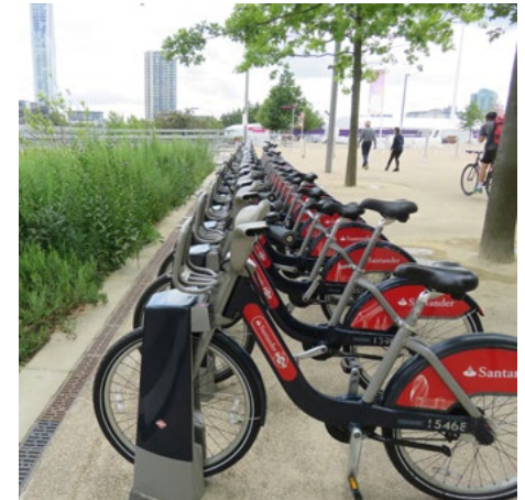
The preferred method of installation with each docking point having an individual concrete foundation; this allows for continuity of surface materials.
