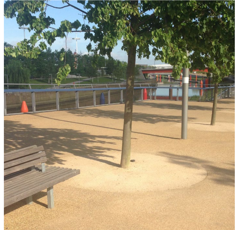
South Park - Tree in a hard landscaped setting with porous CEDEC proprietary gravel
