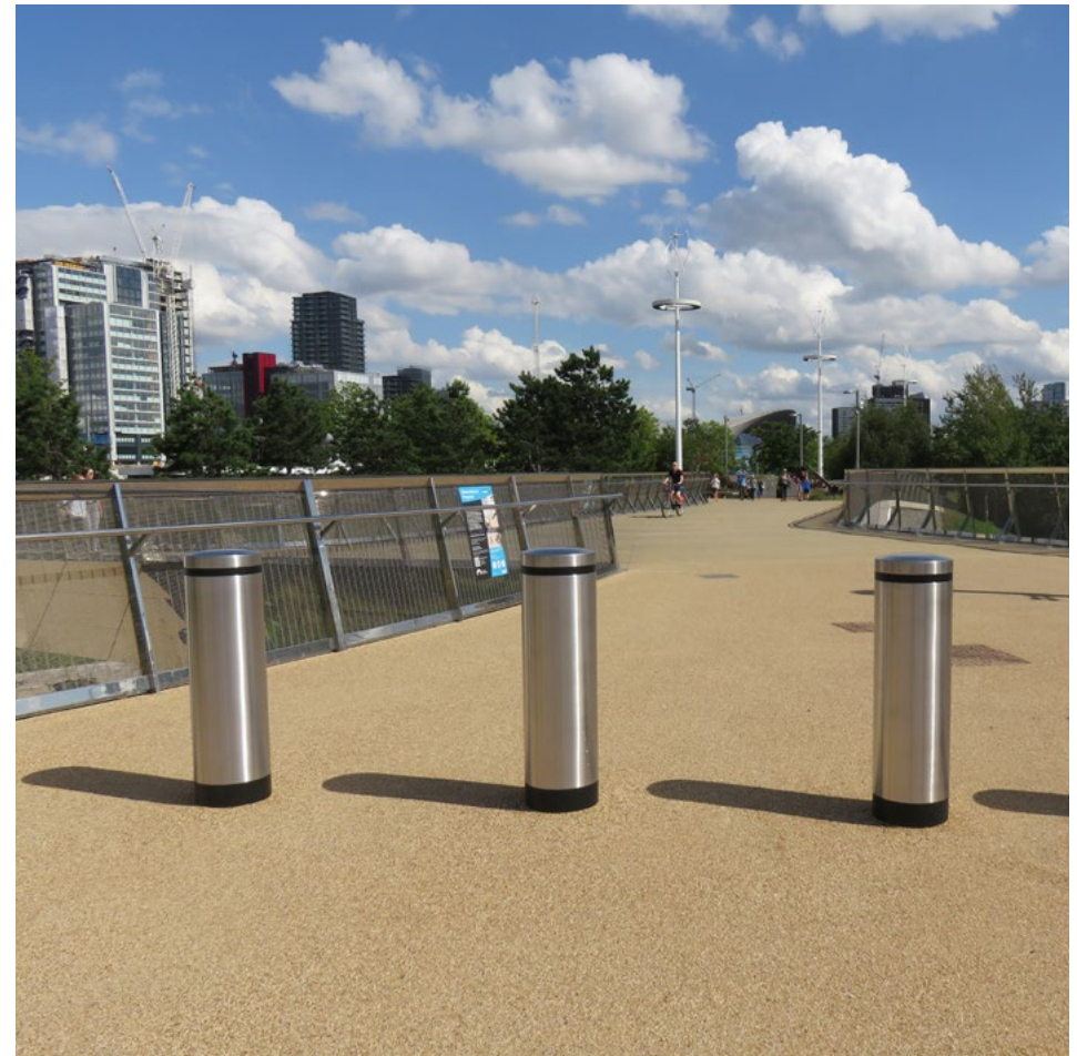
Hostile vehicle mitigation bollards used within the South Park
