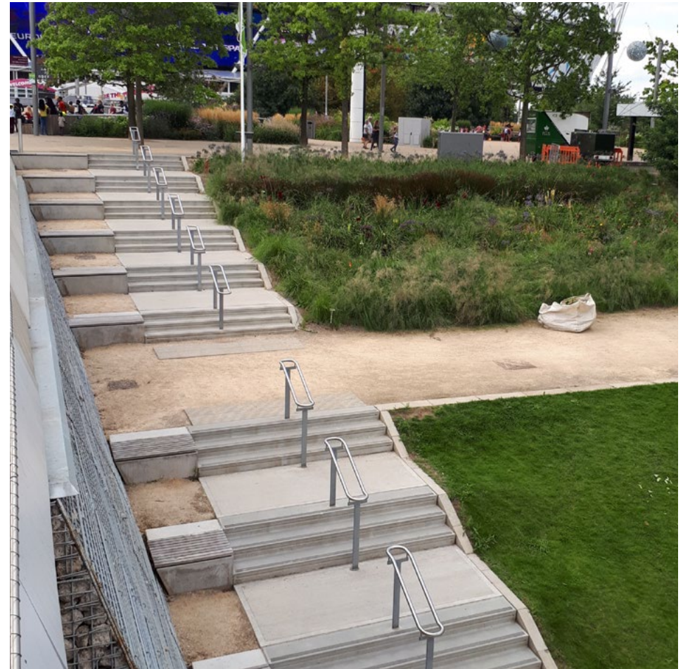
Pre-cast concrete steps with visibility band
