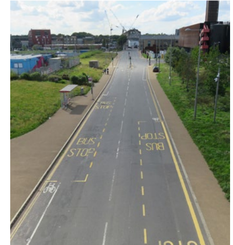
Resin bound aggregate on park edge streets stretch the parkland character out into the wider public realm.
