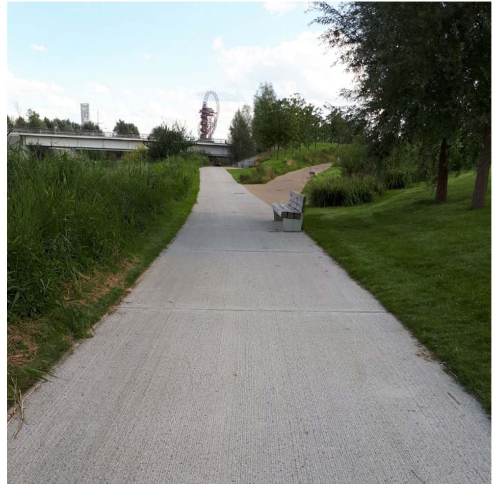
Mechanically scarified concrete in the North Park
