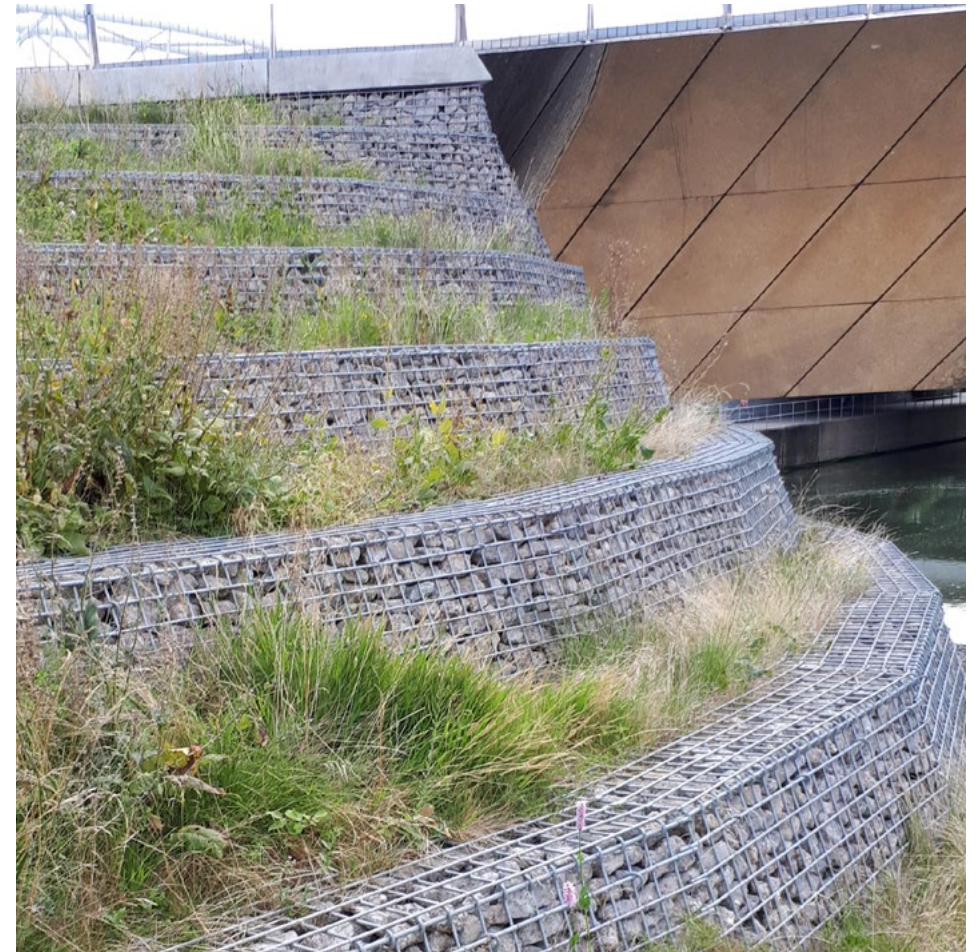
South Park - Vegetated gabion walls
