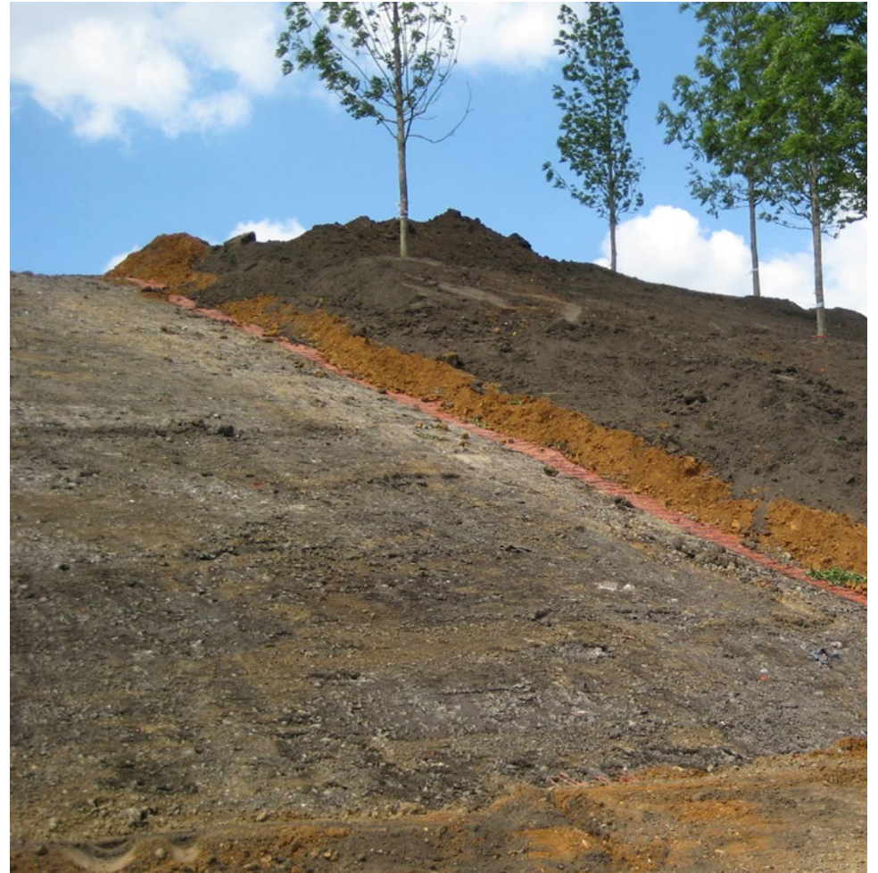
Marker Layer Installation
