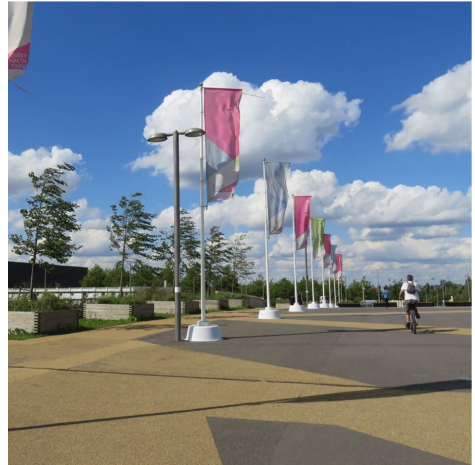
Resin bound gravel and asphalt - South Park
