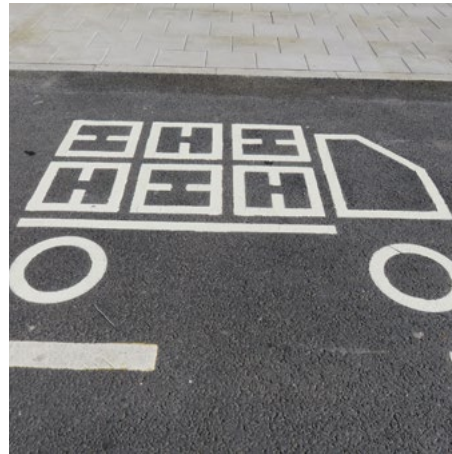
Bespoke surface signage at Here East requires vertical signposts to be legally enforceable.
