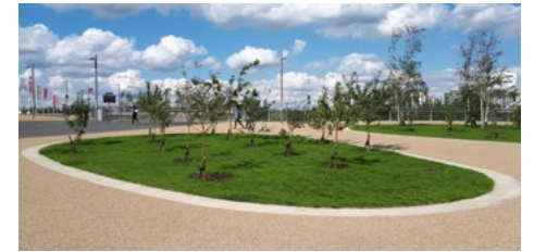
In-situ cast concrete edging - South Park
