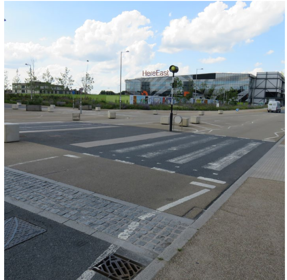
Raised tables and surface materials, help to prioritise pedestrian movements across main roads.
